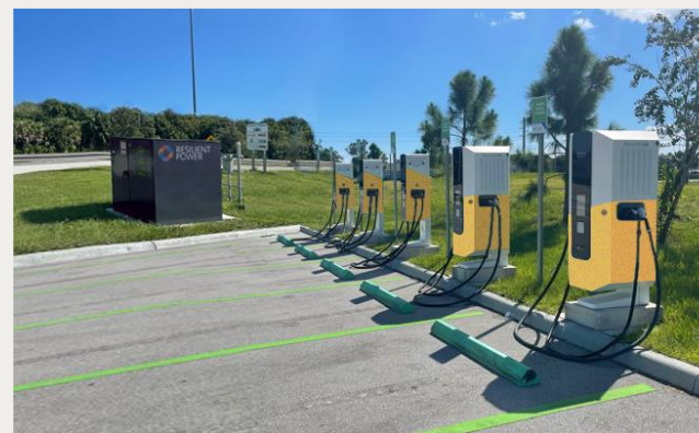
Resilient Power's up to 3.2MW, 15kV 50/60Hz SST (Source: www.resilientpower.com )
