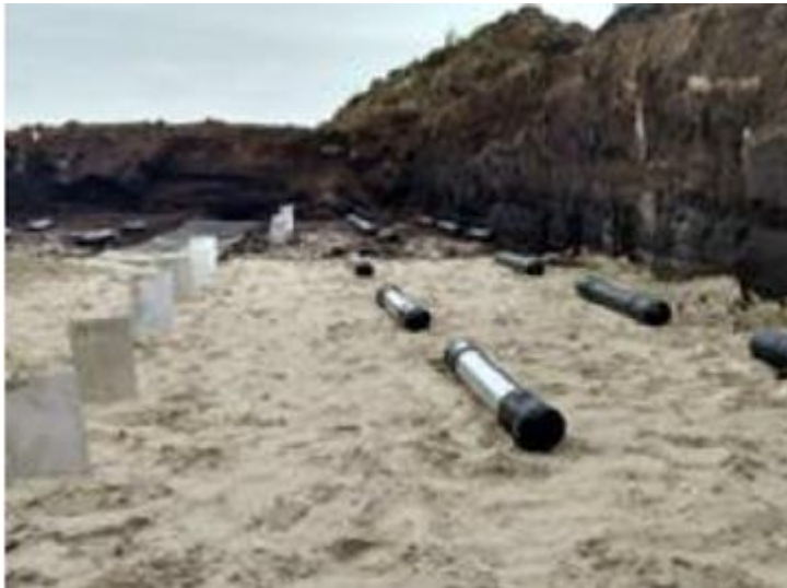
Figure 1 Arrangement of the samples in backfill, before covering and compaction
