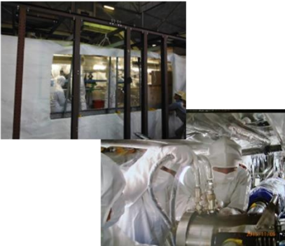
Fig.4 Overview of the verification of premold one piece joint in a narrow manhole
