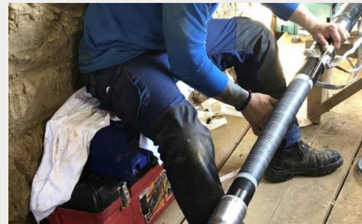
Repair joint installation
