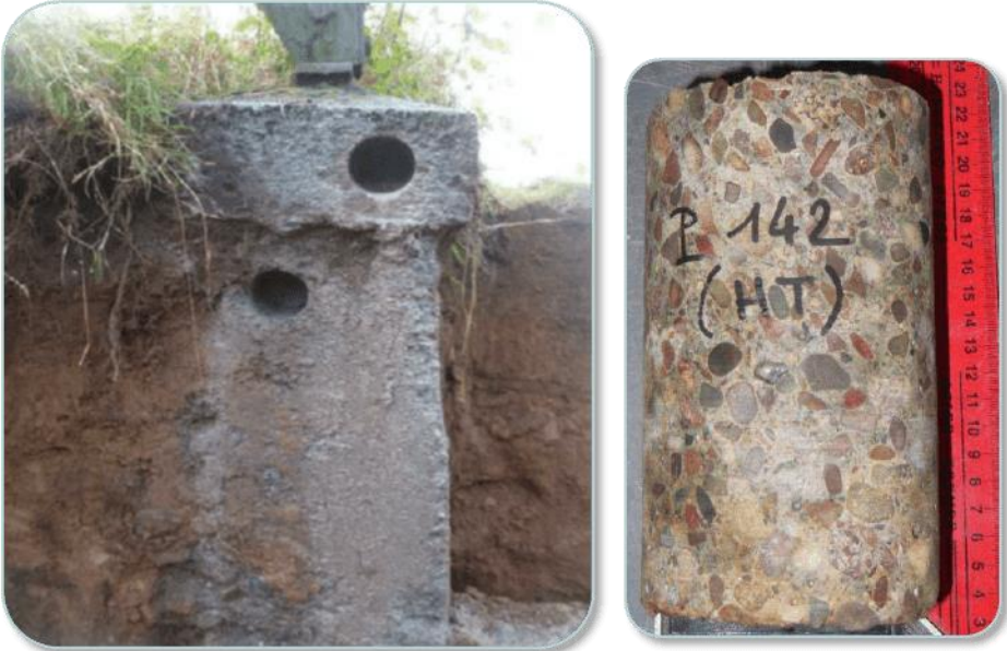
Figure 2 : concrete sampling performed by core drilling on an existing asset
