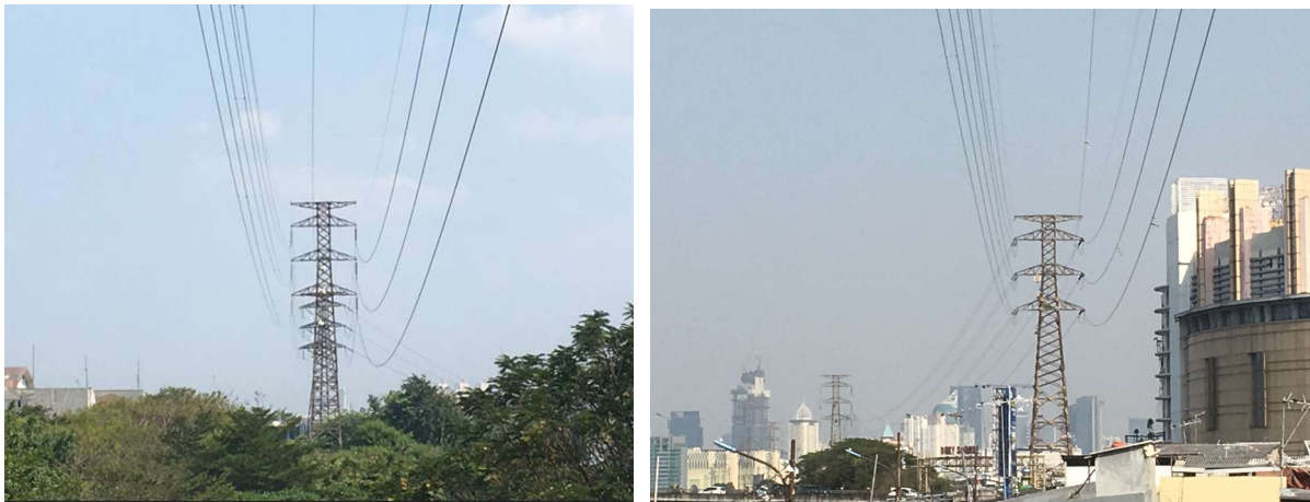
Fig. 2 Comparison of sag at completion of one side line during replacement of ACSR 410 mm 2 single conductor to ACSR 315 mm 2 2 conductor (left side line is ACSR, right side ACSR)
