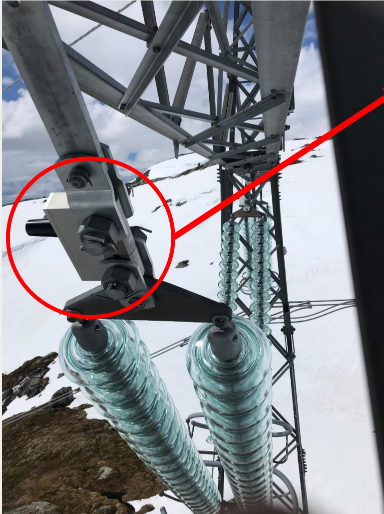
Tension load sensor
