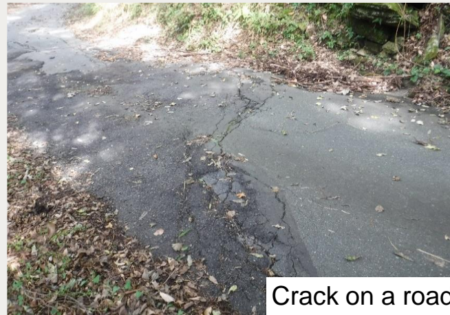
Fig.2 Example of landslide features in field survey
