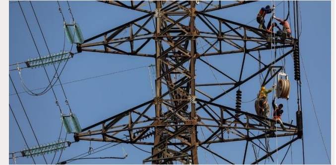
Replacement of ACSR to ACFR
