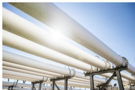
Figure: 420 kV GIL at Richborough UK where first Retrofill was performed
