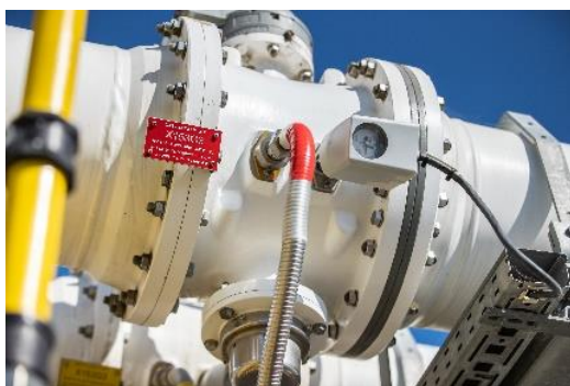
Figure: 420 kV GIL at Richborough UK where first Retrofill was performed
