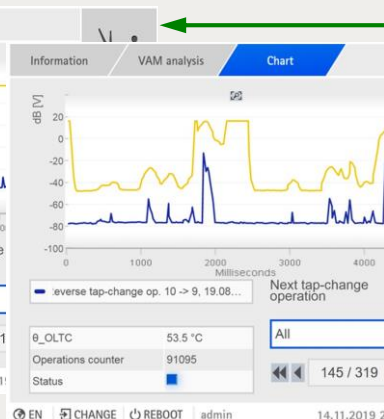
Acoustic envelop after three OLTC operations per tap-changer position
