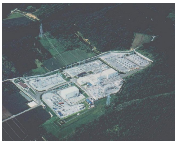
Hakodate converter station
