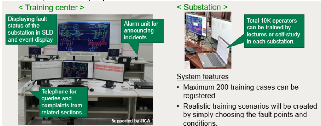
Figure-1 Substation operator training simulators
