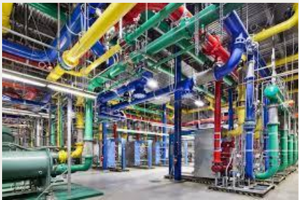
Google data center cooling Partially acceptable
