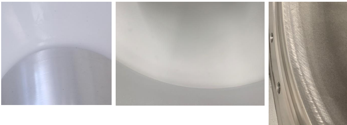
Figure 4. Impressions from visual inspection after thermal aging tests, no solid decomposition products, dielectric tests passed
