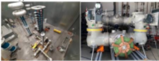
Figure 4.2 – 420 kV GIS device during dielectric test (left) and bus transfer test (right)
