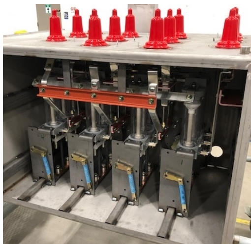
Linear puffer(LP) in switch enclosure
