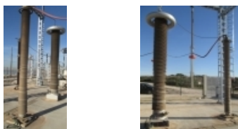
The columns installed in the test area
