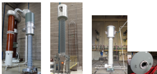
Left and center : Electrical type testing of 420 kV combined and current transformer; Right : 245 kV current transformer during internal arc fault test
