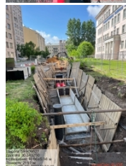
HTS Cable laying
