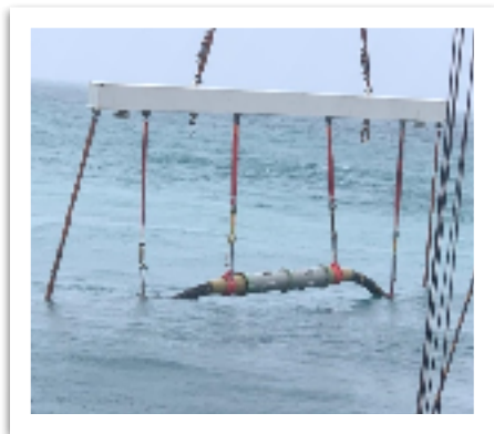
• Figure 7. Completed Joint#3 during laydown to seabed
