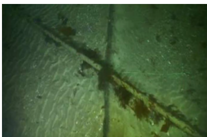
Fig. 7. Power submarine cable crossing with a FO cable
