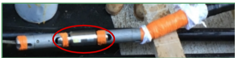
Pulling rope — Swivel — Sensor — Swivel — Head of the cable
