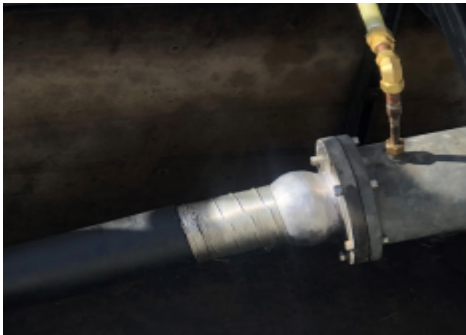
Completed Lead Wipe with Reinforcing Wire and New Fitting
