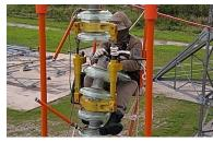
• Tool for replacing a damaged insulator locally in the string
