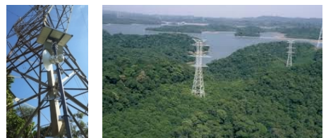
Figure 7 - Challenging in sharing infrastructure of cameras into OHL assets.
