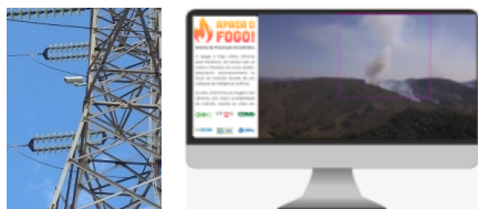
Figure 2 - Video camera on Lattice Tower of 138 kV and webpage interface of algorithms AI system for the detection of fire and smoke interaction with web society.
