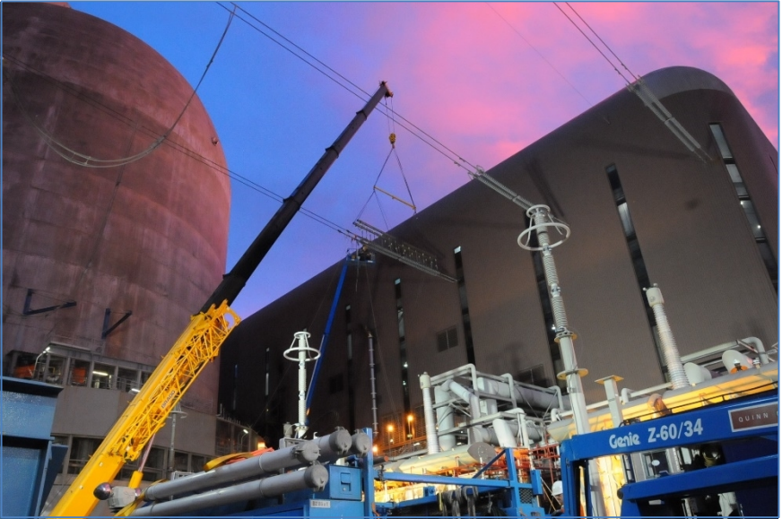
Figure 8: Install of silicone coated glass insulators at Diablo Canyon 2016
