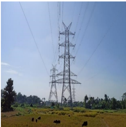
Figure 4: Two D/c lines joining on M/c line
