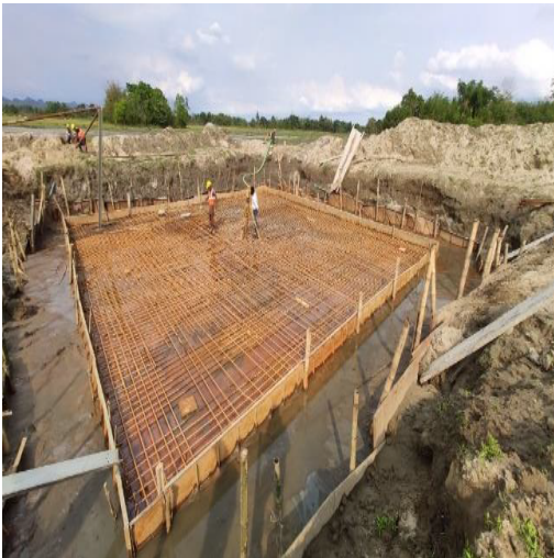
Figure 6: Raft foundation under construction
