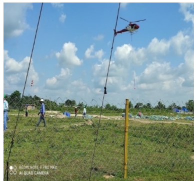
Figure 5: Material lifting using Heli-crane
