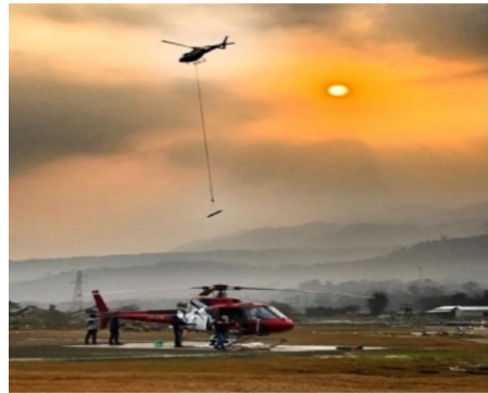
Figure 2: Heli crane operation
