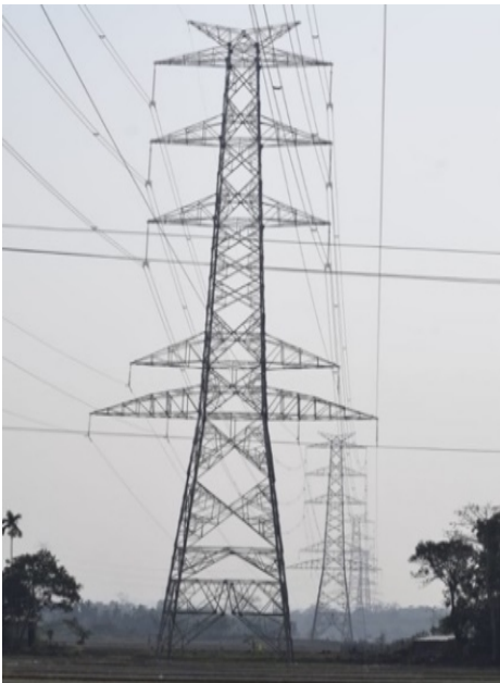
Figure 1: Multi ckt. Multi voltage Line
