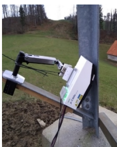
Fig. 3 Measurement of initial stress in legs of towers
