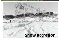
Fig. 1 Tower collapses and damages
