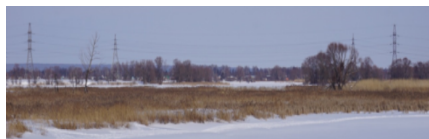
Fig.1. Photo of the span with supports, date 05.03.2021
