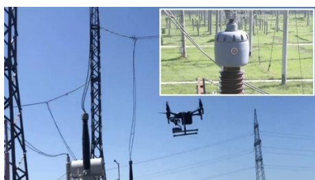
Location of cameras of the visual monitoring system on the auto transformer.
