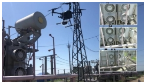
Inspection of the substation using UAV
