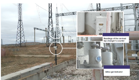
Location of cameras of the visual monitoring system on the auto transformer.
