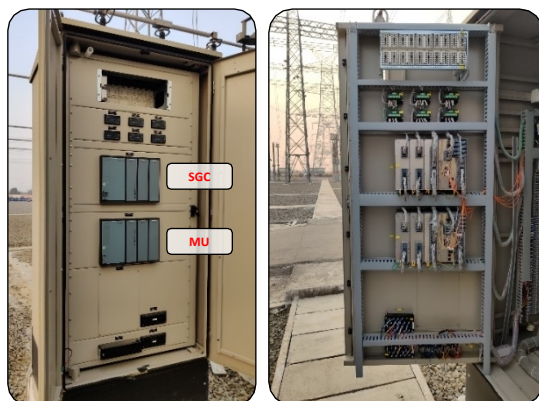
Figure 3-Marshalling Boxes housing MUs & SGCs
