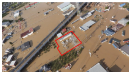
Fig. 2. Picture of substation flooding
