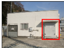
Fig. 15. Watertight door of the main building
