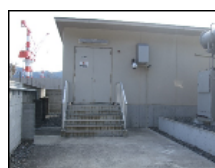
Fig. 13. Raising floor level of a main building
