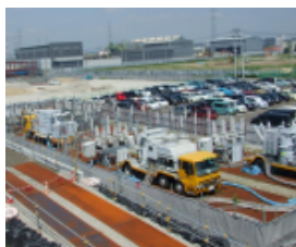
Fig. 9. Mobile substation
