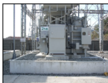
Fig. 12. Raising foundation level of transformers
