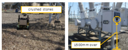
Fig.1. Crushed stone ground and Inspection window height
