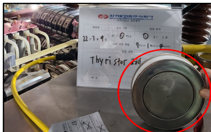
Figure-3 Photo at the time of replacement Thyristor
