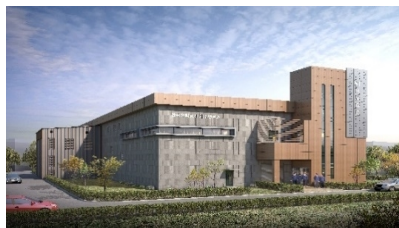
Figure-1 #1 HVDC Converter Station
