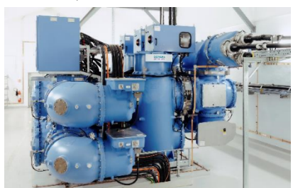
Clean Air Vacuum GIS 145 kV / 40 kA / 3150 A / -50°C / 1g
