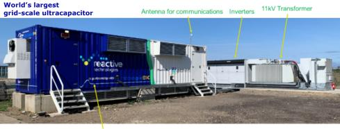
Container houses ultracapacitor cells and modules, control system, cooling system, fire detection and suppression
