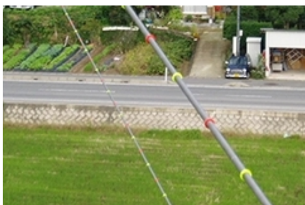
Fig. 3. Example of the Ring-type diverters (Image courtesy of Kansai Transmission and Distribution, Inc.)
