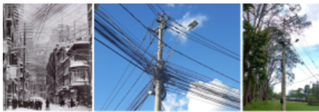
Figure 1 - A critical view of the concept of Synergic Networks: (a) the old problem of sharing cables on poles, (b) the sharing problem persists and (c) the new topology proposed for Synergic Networks in test at UniverCemig.
