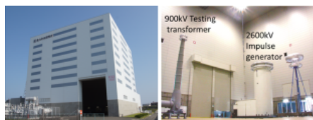
(a) Exterior (b) Power supplies Figure 4. High voltage laboratory of CRIEPI
