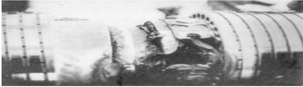
Figure 1. Shaft damage at Mohave power plant [2]
