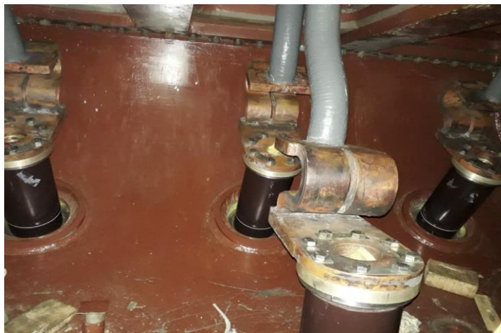
Fig.2 Detailed view of flexible droppers from CBBs to Bushings.
