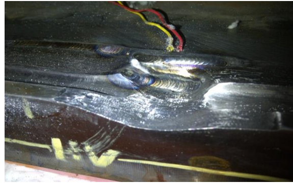
Figure 20. Slot 11 ready for weld repair
