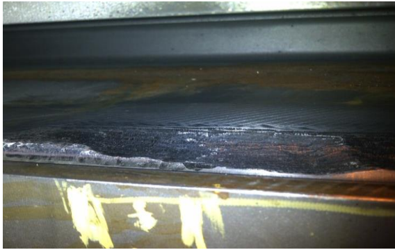
Figure 19. Slot 24 ready for weld repair
