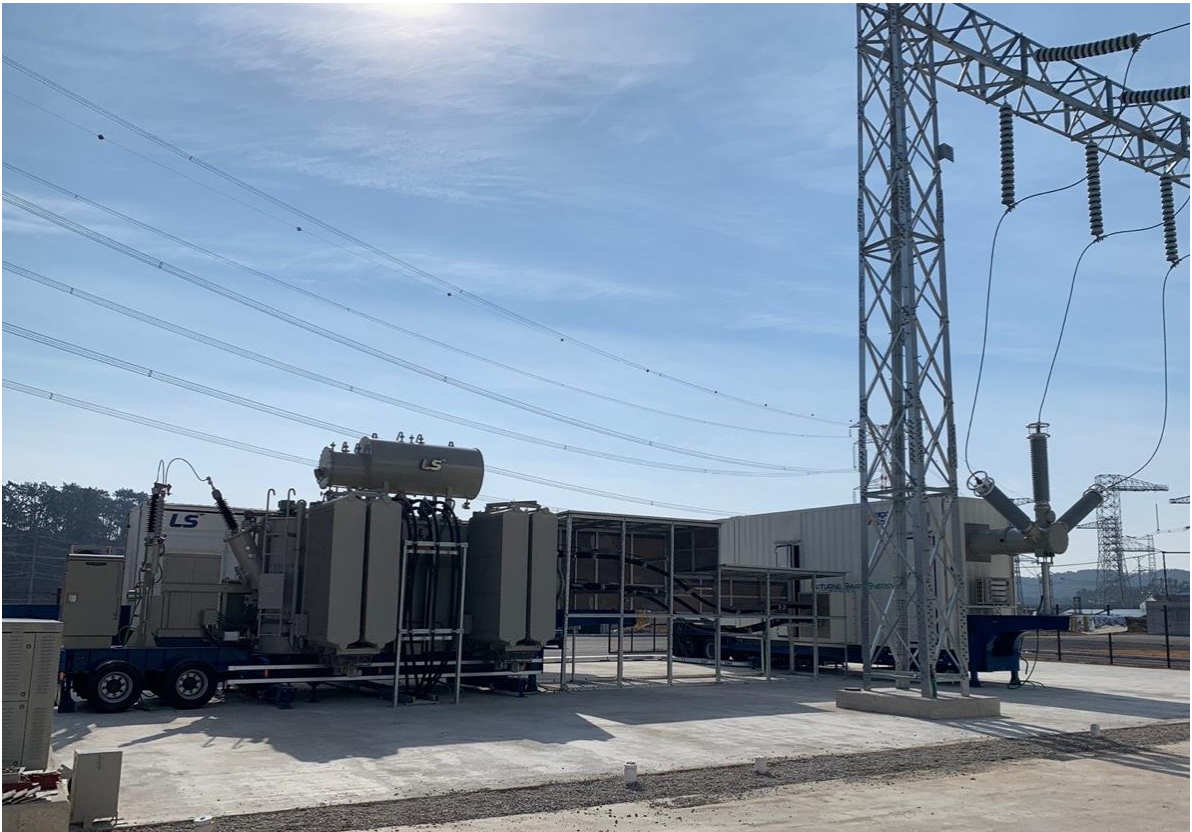
Figure 12 – Installation of modular type equipment for pilot test
