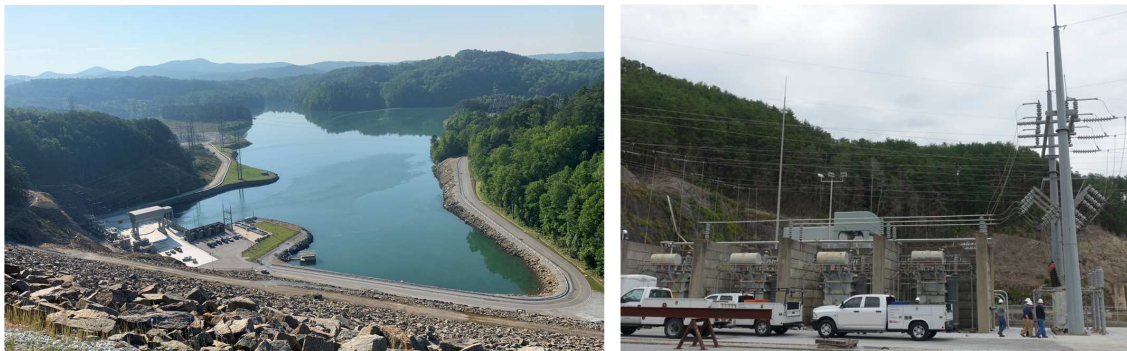
Fig. 6 – Hydroelectric power station where the first 145 kV dry-type transformer was installed: overall view (left); fifty years old three-phase bank to be replaced (right)
