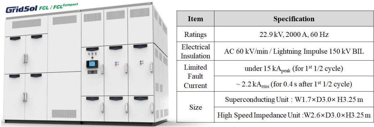
Figure 1. Appearance and specifications of a 22.9 kV/2.0 kA R-SFCL
