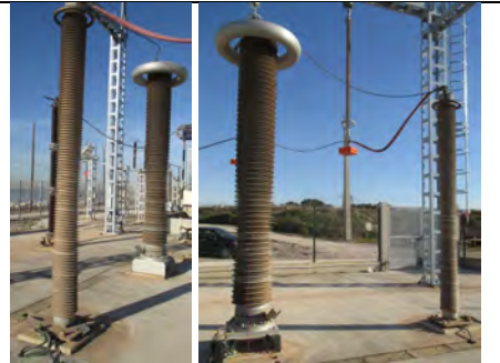
Figure 9b: The columns installed in the test area
