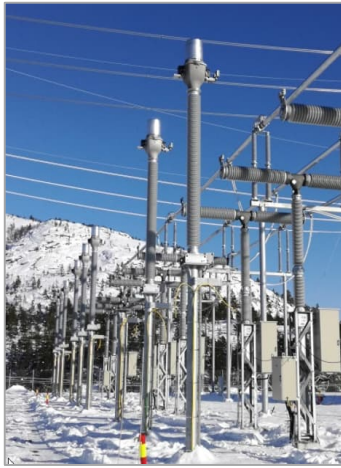
Figure 11: High Voltage oil Current Transformer installed and sectional view (top cores design)
