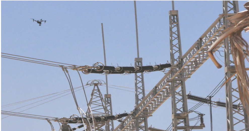
Figure 7: UAV over Live EHV circuits
